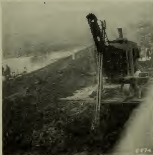
STEAM SHOVEL CUTTING DRAINAGE TRENCH.
